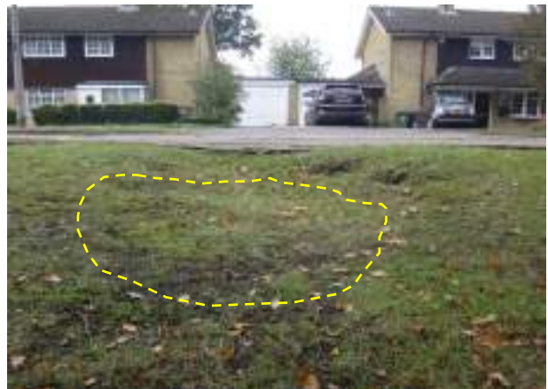
Area of ground subsidence in grass verge highlighted in yellow.
