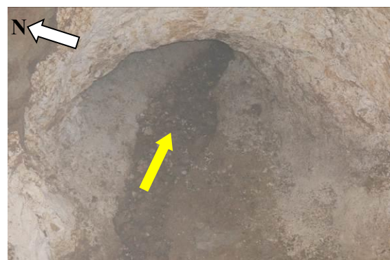
Plate 9 – (Top) General image showing the tunnel location at the base of the void. (Below) Close up of assumed tunnel.
