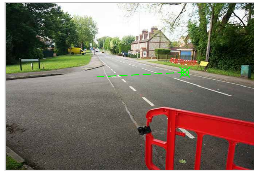
P1a: GENERAL VIEW OF ROAD AT BRANKSOME CLOSE JUNCTION LOOKING NORTH - ZERO DATUM INDICATED
