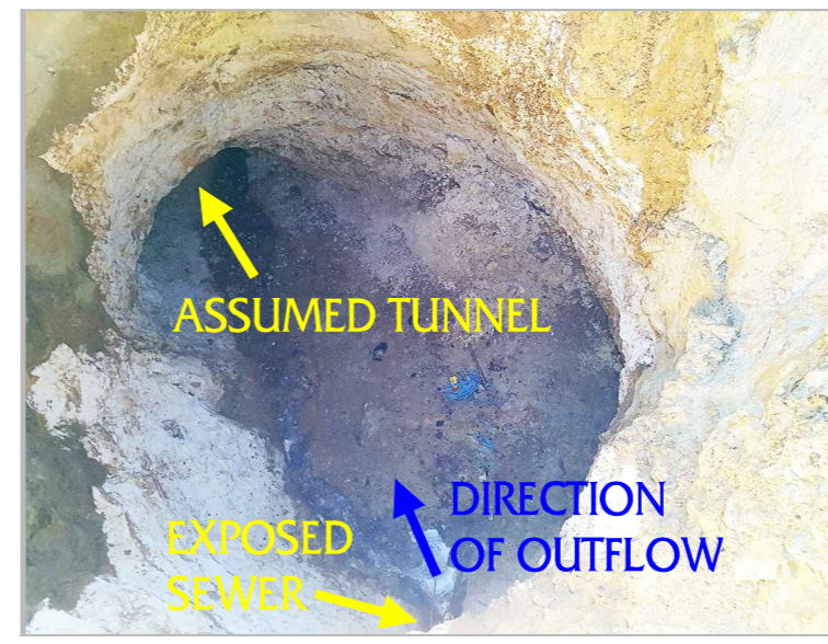
P2b: VIEW INSIDE 'VOID' LOOKING SOUTH EAST
