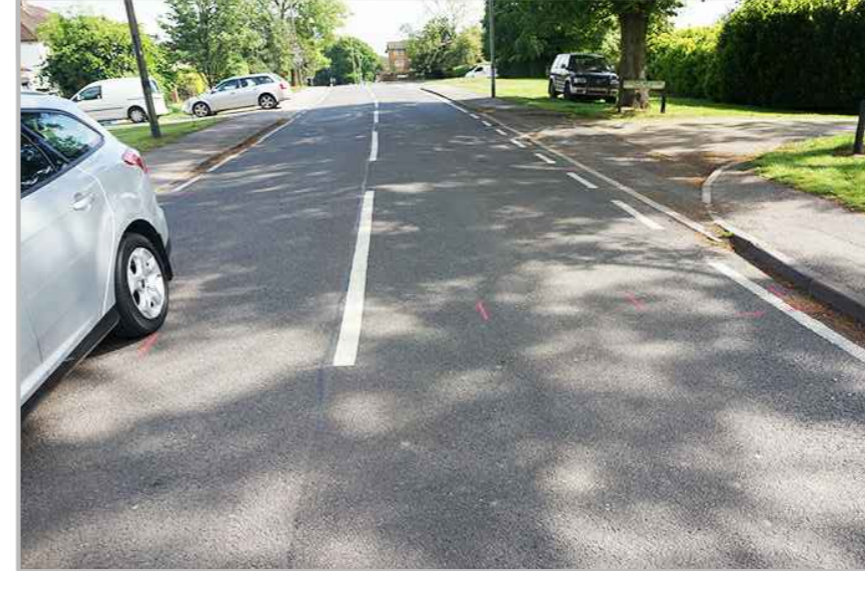
P1b: GENERAL VIEW OF HIGH STREET GREEN LOOKING SOUTH
