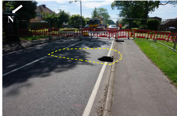
Plate 6 – Approximate extent of void marked on surface by GBG.
